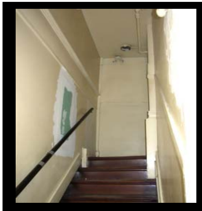
Repairs Being Made to a SRO Hotel Hallway
