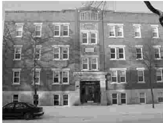
Fig. 5.2. Trevere Apartments, 300 Furby Street, built 1926
