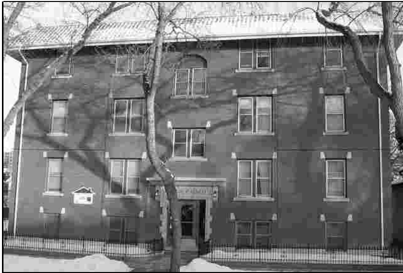
Fig. 3.1. The Cambridge Apartments, 303 Furby Street, built 1926
