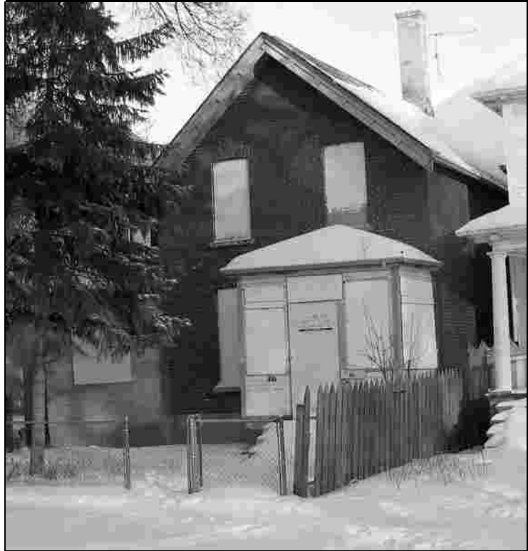
Fig. 3.7. The Correia home, 297 Furby Street
