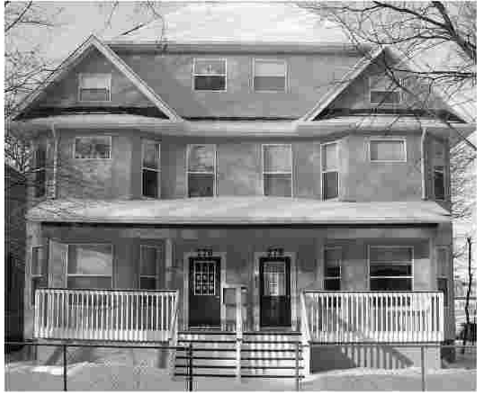
Fig. 4.4. 276/278 Furby Street after renovations
