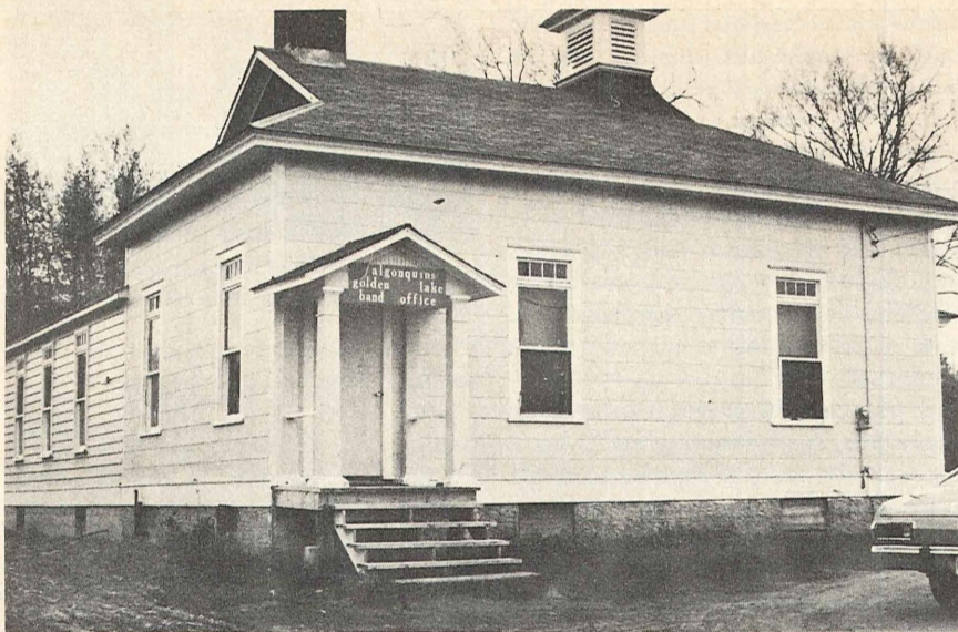
The old federal school building and now a Band Council Hall which the band council hopes to move out from soon, leaving it free for other uses.
