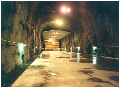
"Forsmark Horizontal silo" by Fred Dawson is licensed under CC BY-NC-ND 2.0
