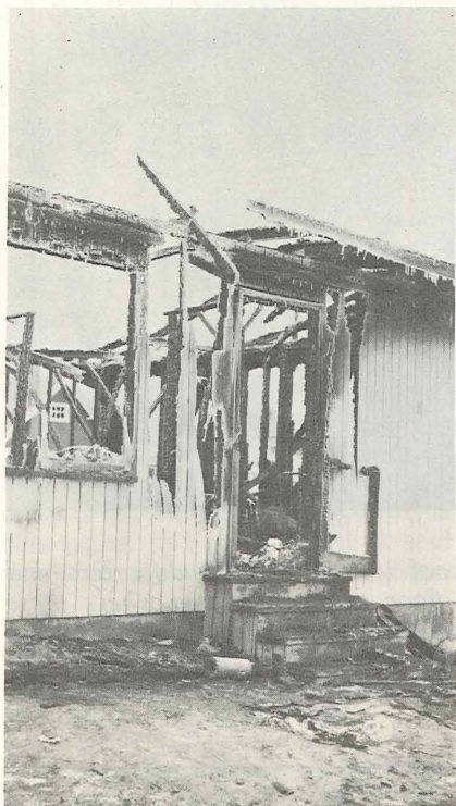
A front view of the home where seven children died. This door was blocked and what could have served as an exit became a death trap.
