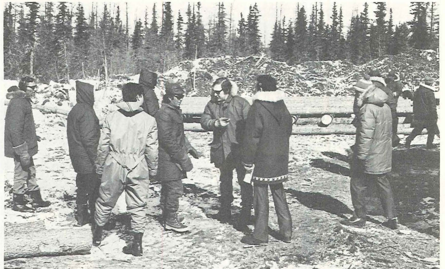
Technical Services civil engineer Gary Epps, explains to construction crew how materials will be arriving at James Bay Reserve during spring breakup.
