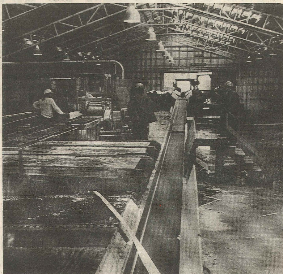
Just enough room for the equipment? Wrong, says Willie Wilson. Close to 50 per cent of the floor space in the main mill shed is available for additional equipment. "Actually, we have only half a mill," he says. "But since creating more jobs at the Reserve hinges on doing more with the lumber we produce rather than producing more lumber, there is no need at the present time to enlarge the mill or add significantly to our production capacity."
