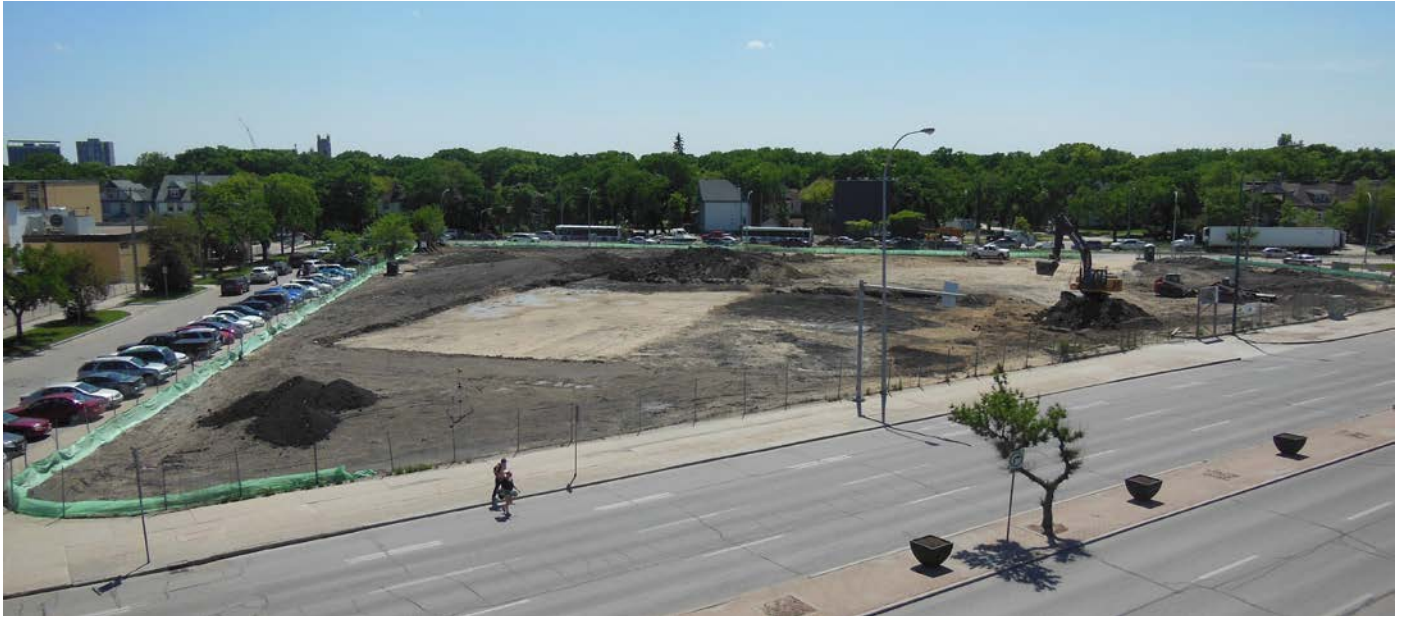
The proposed greenspace under construction, spring 2012.
