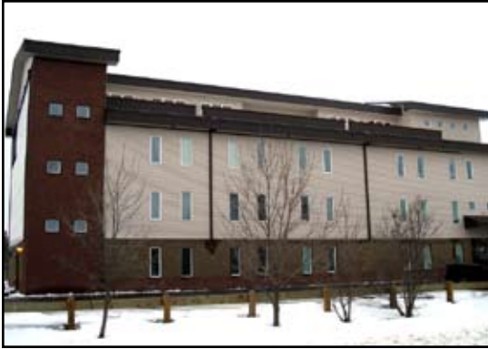
An assisted living facility in Arborg; there is great demand for similar projects in all areas of the East Interlake.
