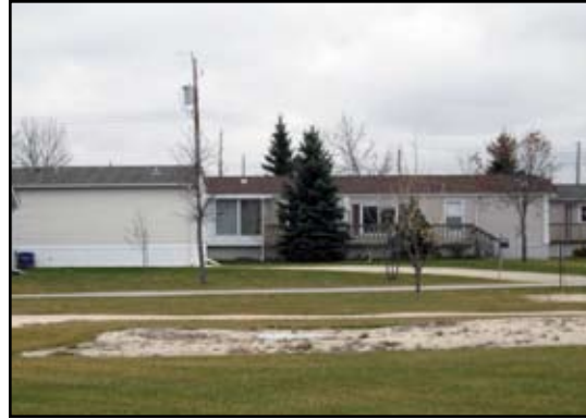
Crescent Creek Modular Home Park in Teulon, owned and operated by the municipality. All Photos: Kaeley Wiseman
