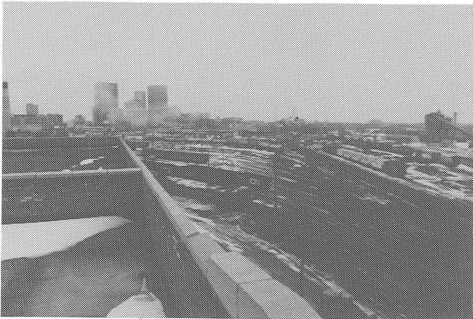
Illustration 4. Empty sidings, rusting trackage at the heart of the former freight marshalling yards.
