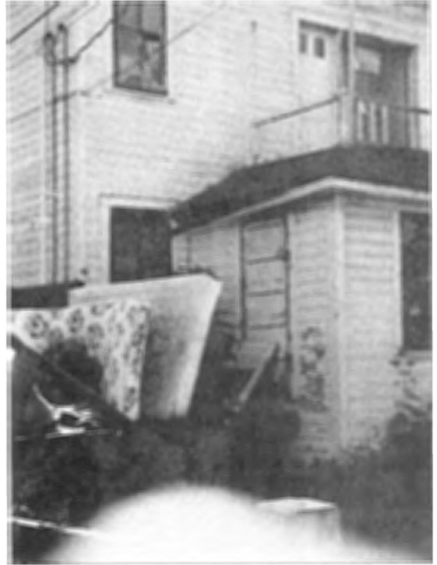
↑ Dilapidated Housing on Spence Street
