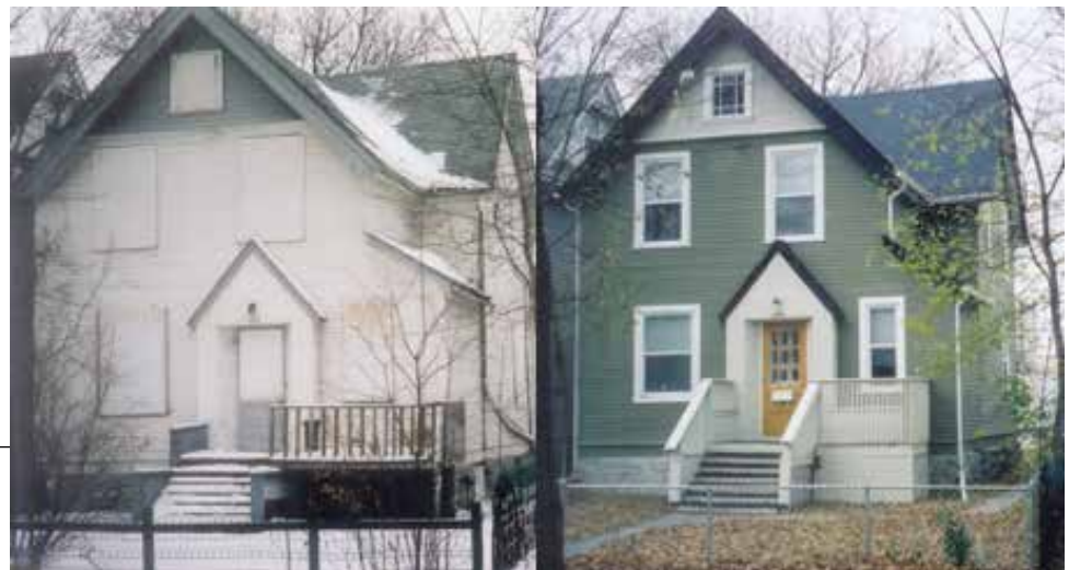
Westminster Housing Society Early Renovation Project— Before and After.
