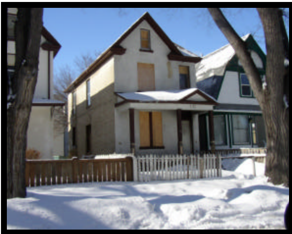
House in need of major repair
