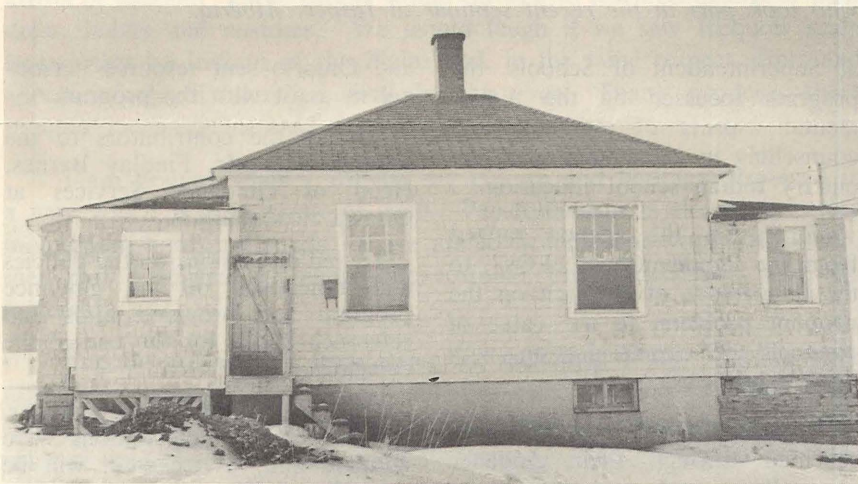
BEFORE — A side view of Mrs. Mary Ann Goulds' home prior to reconstruction. Many of these homes were erected 40 years ago.
