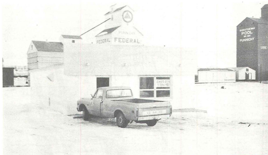
A clean, bright-looking building the laundry, shown from the outside, displays a welcome sign in its window, "Always ready to serve you".
