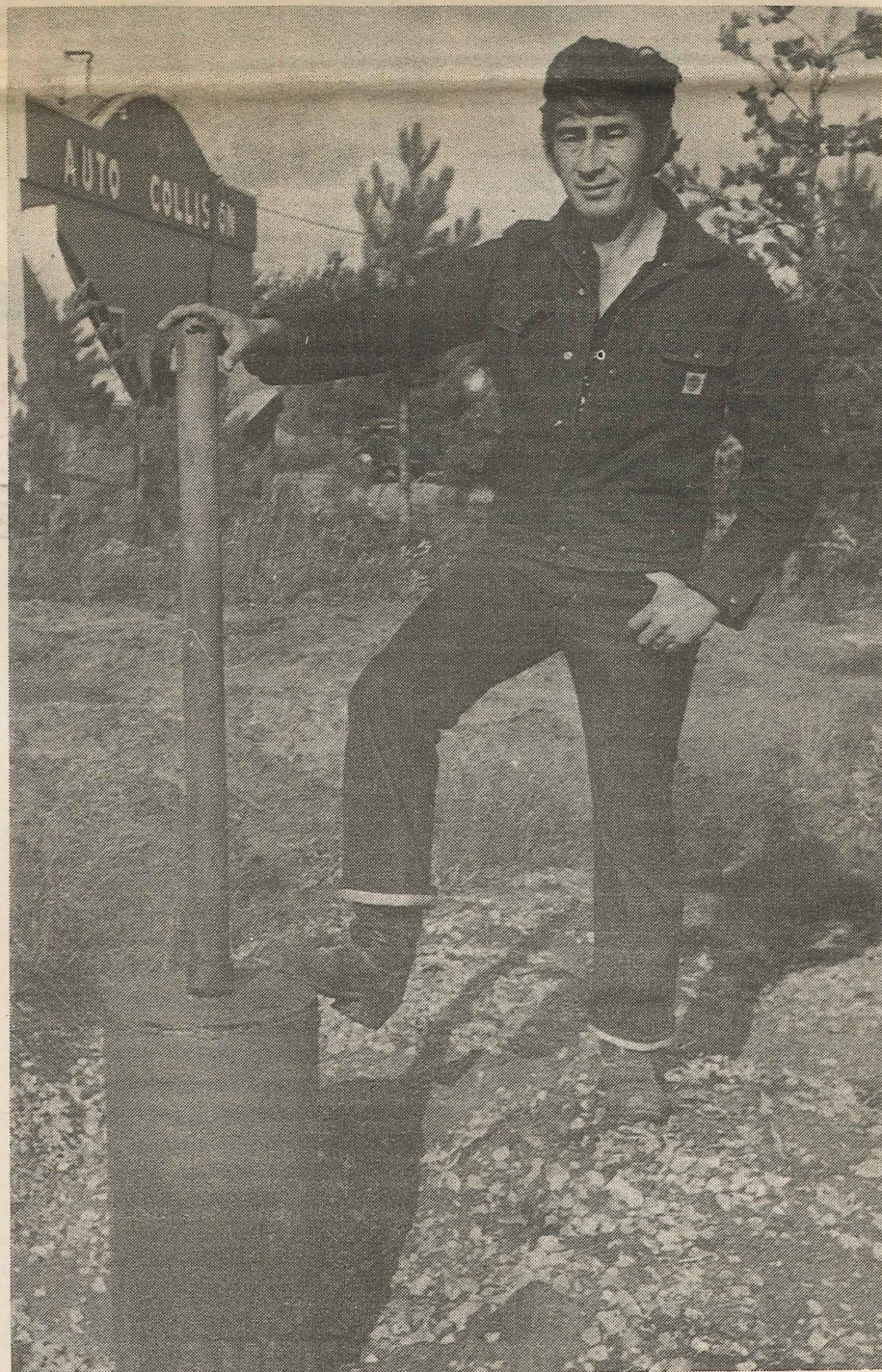
Rankin Reserve Chief John "Duke" Corbiere points to the deep well drilled in the Reserve's industrial park. The modern pumphouse over the well will mean full servicing for the eight industries which have already located in the park. Behind the Chief is a body repair shop, a pioneer industry at the site.
