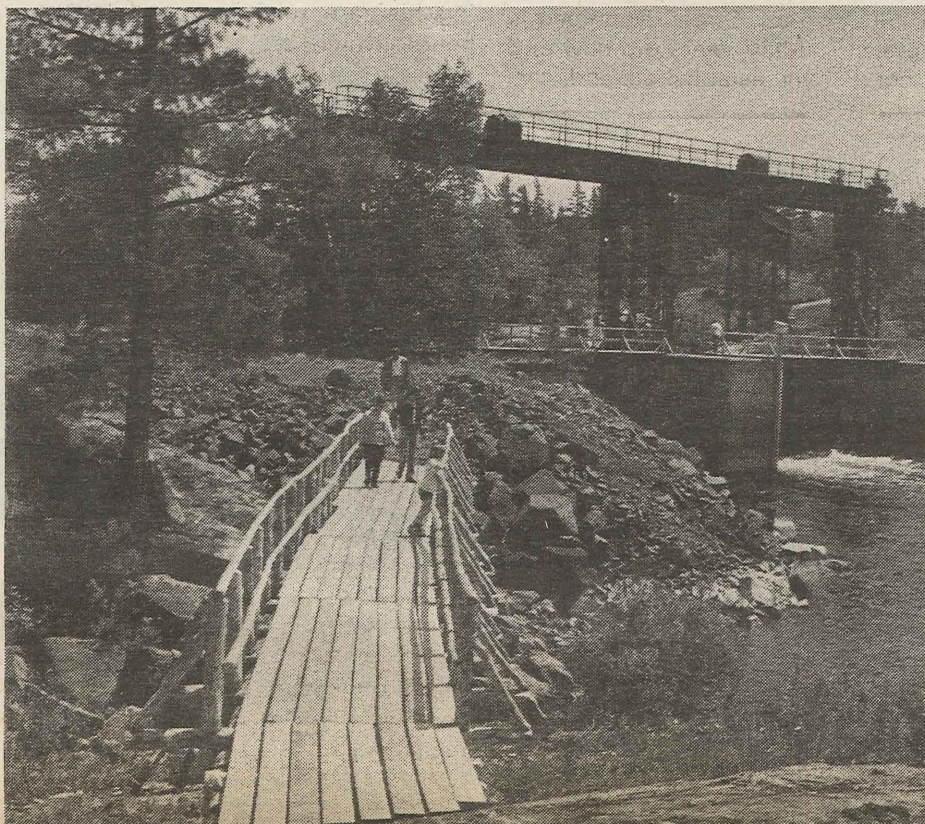
The trails to the Chaudiere Dams on the French River are bridged by structures such as these, using logs and rough lumber.
