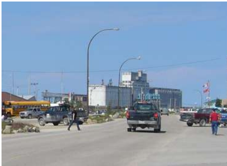
Churchill's Grain Elevator From Kelsy Blvd. Picture by Fereshteh Moradzadeh
