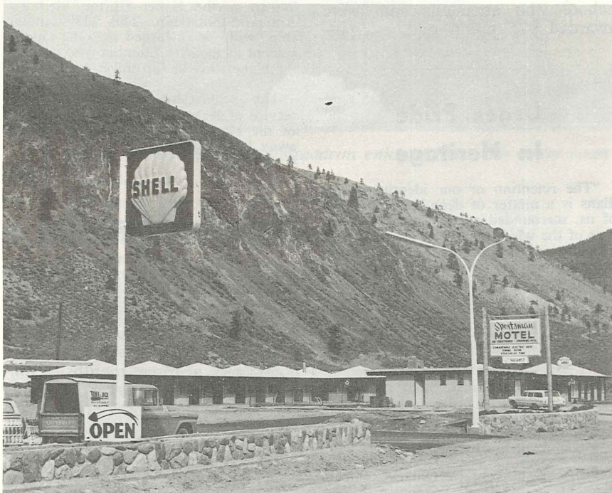
Above is the Sportsman Motel which is a joint enterprise of the Walkem family, Spences Bridge, British Columbia.
